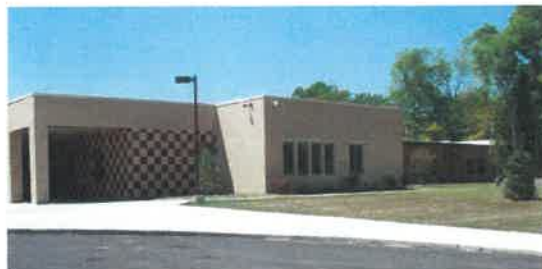
Westbrooke Village Elementary School
